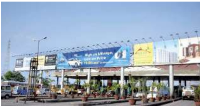
Dahisar toll plaza
