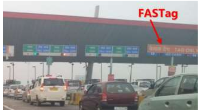
Vashi toll plaza
