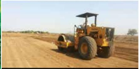
Work in progress at embankment top layer
